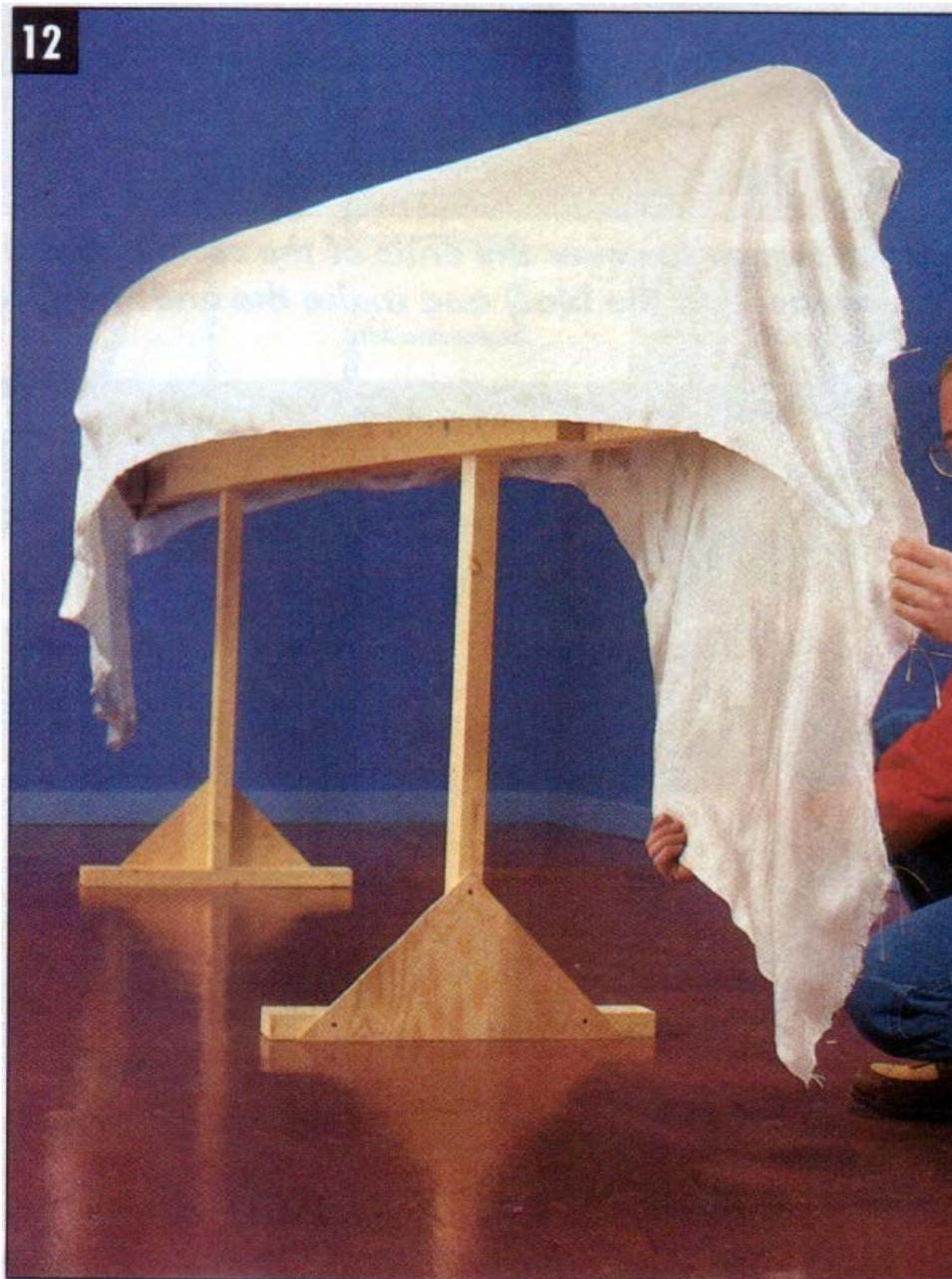
**LAY FIBERGLASS** cloth over the hull so the weave is at an angle to the keel, then trim off the overhanging pieces. Trim the cloth an inch or so short of the ends of the canoe.
