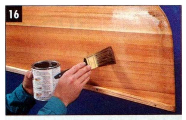
APPLY TWO COATS of clear exterior polyurethane to the hull and to all the ash trim. Then break out the paddles — you're finished!
