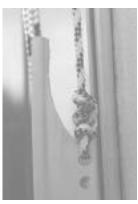
Hoist the profile by means of a flag-line in the top. Use therefore the upper-hole in the plastic profile.
